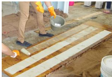
a. Applying epoxy to GFRP
