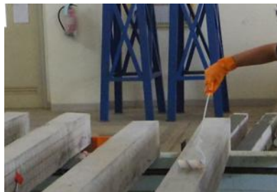
b. Impregnation of epoxy
