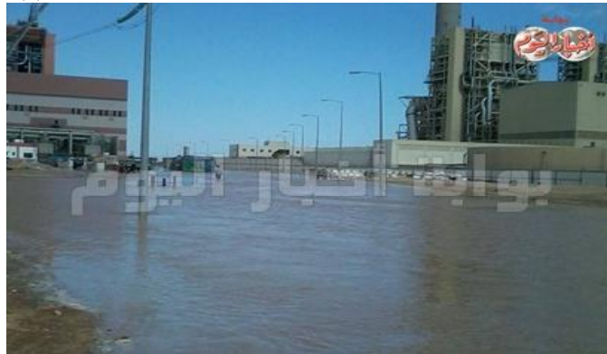
Fig (1): Flood in El Ain El Sokhana Power Plant, 16, May 2014, [9].
