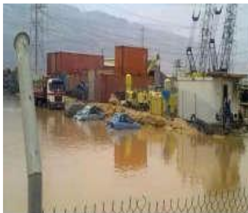
Fig (3): Damage of cars and Equipment during Flood inside the El Ain Al Sokhana Power Plant, 16, May 2014, [9].
