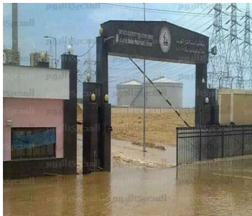
Fig (2): Flood in El Ain El Sokhana Power Plant, 16, May 2014, [9].
