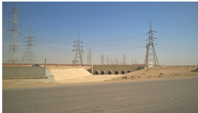
Fig (5): New Flood Culver introduced as an Engineering Solution to reduce Flood Risk in El Ain El Sokhana Power Plant, Photo by the Author.
