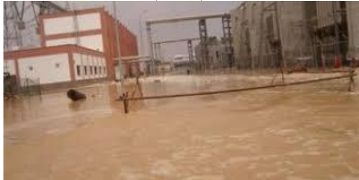
Fig (4): Flood in El Ain El Sokhana Power Plant, 16, May 2014, [9].
