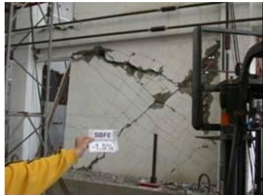
Photo 4. The wall damaged severely at 1.5% drift
