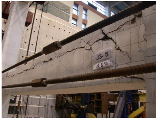
Photo 1. The major cracking on the top of the beam
