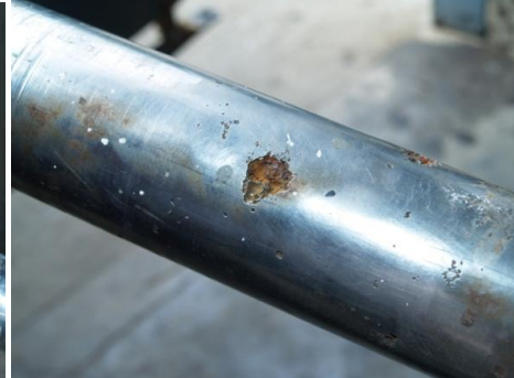
Fig.4. Deep pitting on bearing area
