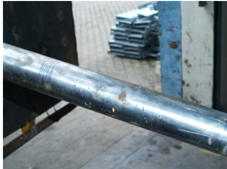
Fig.3. Corrosion in propeller shaft
