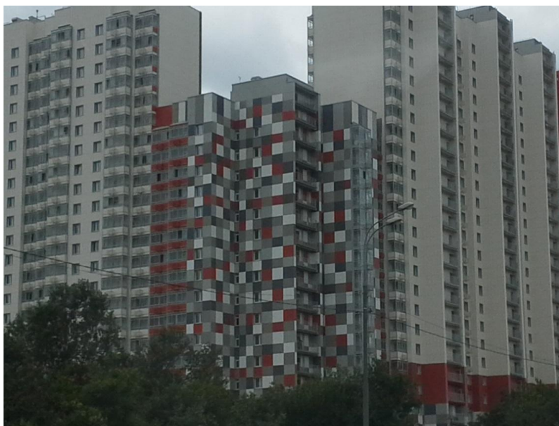
Pic.5 An interesting example of rehabilitation of the residential district in Moscow; The „corner” is easy do identify and in fact became a „landmark”, author: Felski B.
