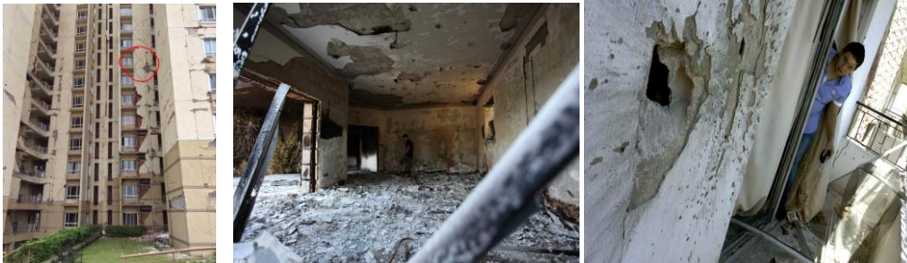
Fig. 1. The destruction of buildings in Libya
