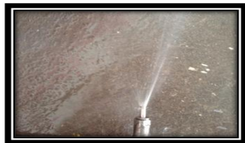
FIG -13. 3HOLE NOZZEL Z TYPE RETROFIT WITH HOLES
