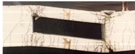
Fig (4). Ductile failure of a beam under combined bending and shear.
