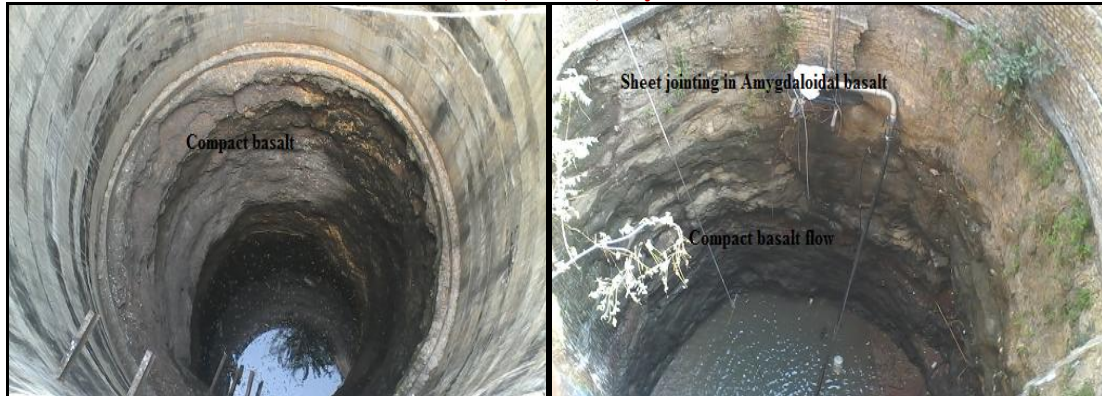
Fig. 5: Dug well in the Contact basalt Flow at Dharmapuri village basalt at Dharmapuri
