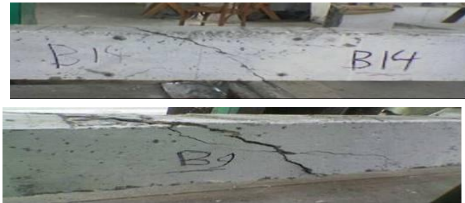
Fig 5. Crack Patterns and Failure Modes Of Some Specimens
