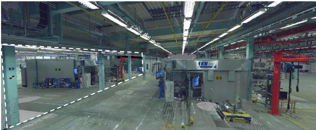
Fig. 4: Point cloud of proposed layout, future layout outlined on the left hand side
