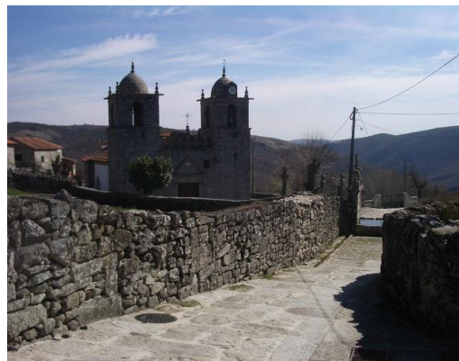
Fig. 4. Access to the Church
