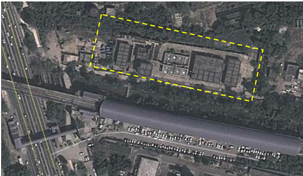
Fig.1 Satellite image of STP based on BIOFOR Technology at Sen Nursing Home, Delhi (Acquired from Google Earth)
